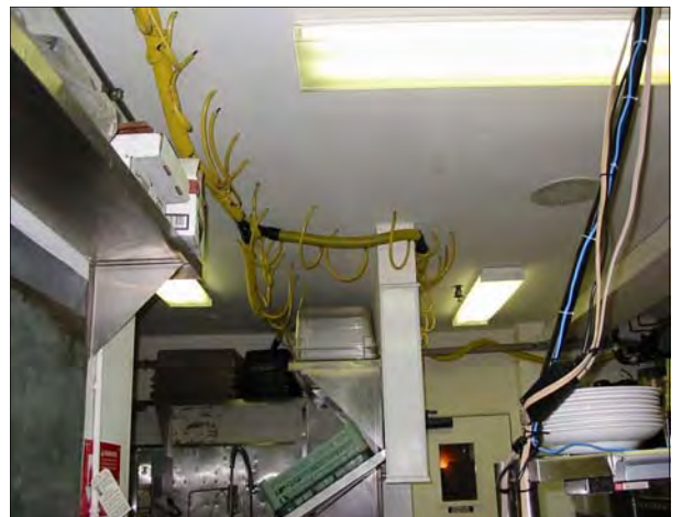
Wall drying behind tile
