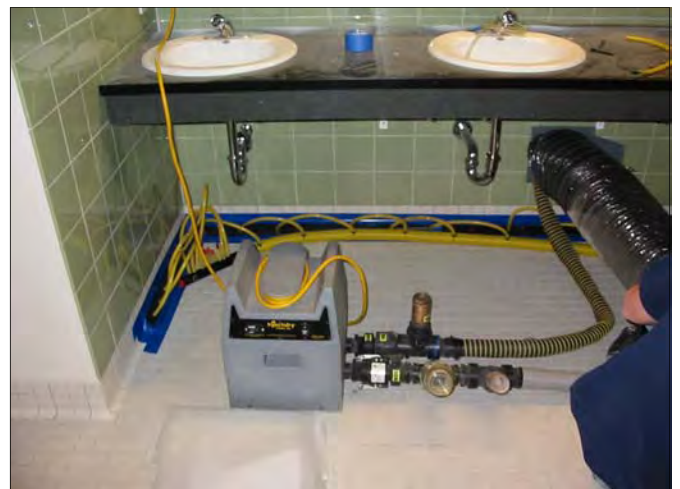
Wall drying behind tile
