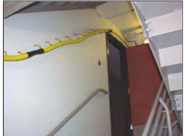
Ceiling and wall dryouts using the INJ01 with patented Active Hoseline (tubing can be cut to the length needed for the job)
