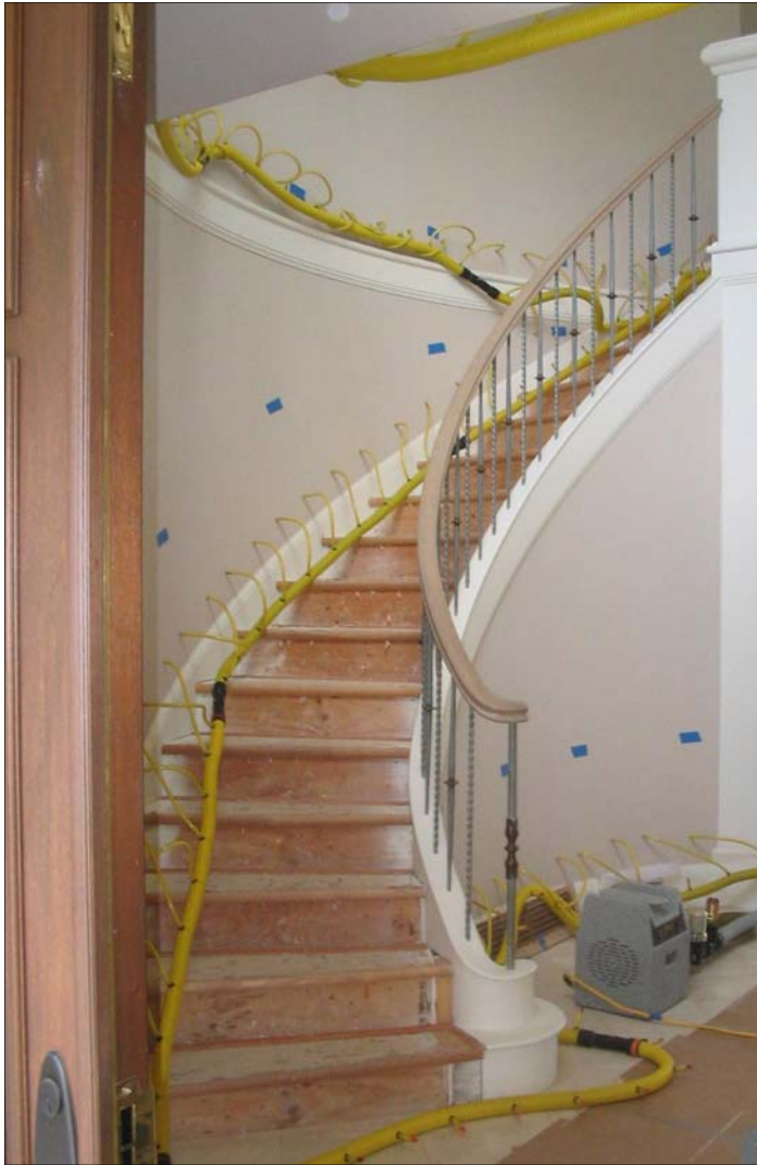
Ceiling and wall dryouts using the INJ01i with patented Active Hoseline (tubing can be cut to the length needed for the job)
