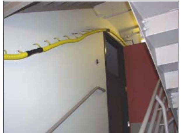
Ceiling and wall dryouts using the INJ01i with patented Active Hoseline (tubing can be cut to the length needed for the job)
