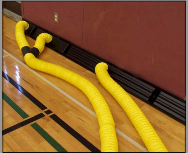
Closeup of wall vents
