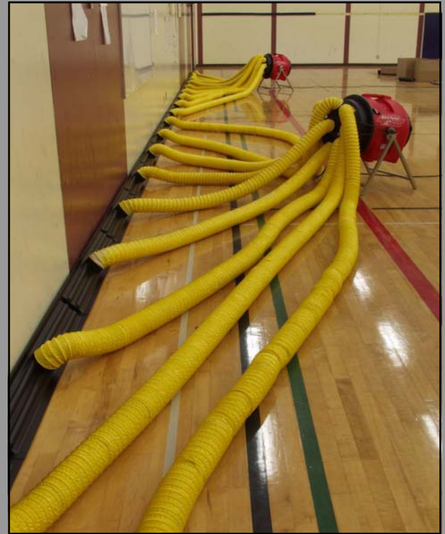
ADP9 on MAX Forces drying a sleepered floor system
